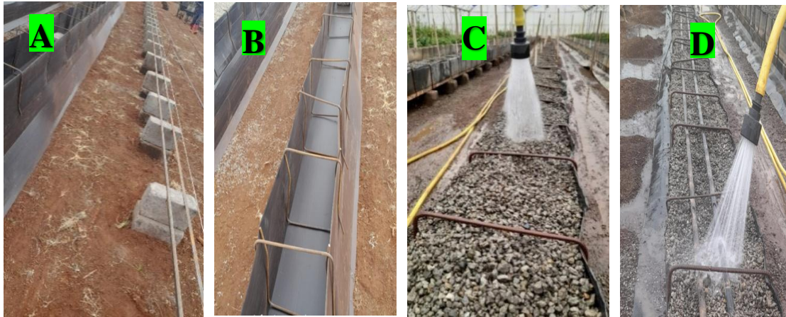
Plate 1: Raising of Hydroponics Planting Beds (A), Reinforcing the Planting Troughs (B), Sterilizing the Media with Hydrogen Peroxide (C) and Stabilizing Planting Media pH with Phosphoric Acid (D).
