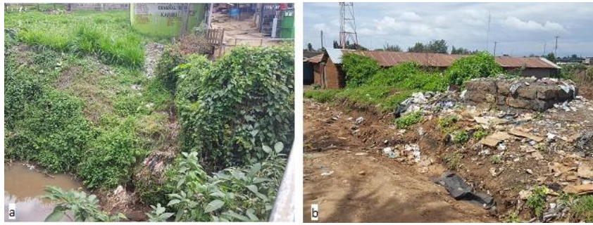
Plate 2. A waste dump with waste overflowing to a nearby river (a) and an improved waste pit with raised stone walls (b) at Njokerio centre
