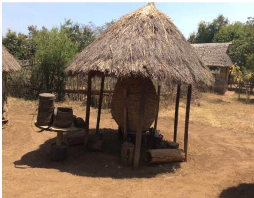
Plate 3 : Granary made of hurdles-work of thin bendable rods (Ikumbi ria Ndi) found constructed at in Josphat Waikwa's homestead at Kamangu-Kikuyu (top) photo taken on 22rd June 2017, and granary (bottom) made of woven grass into a porous basket, constructed at Thingira cultural center photo taken on 3 rd February 2019.
